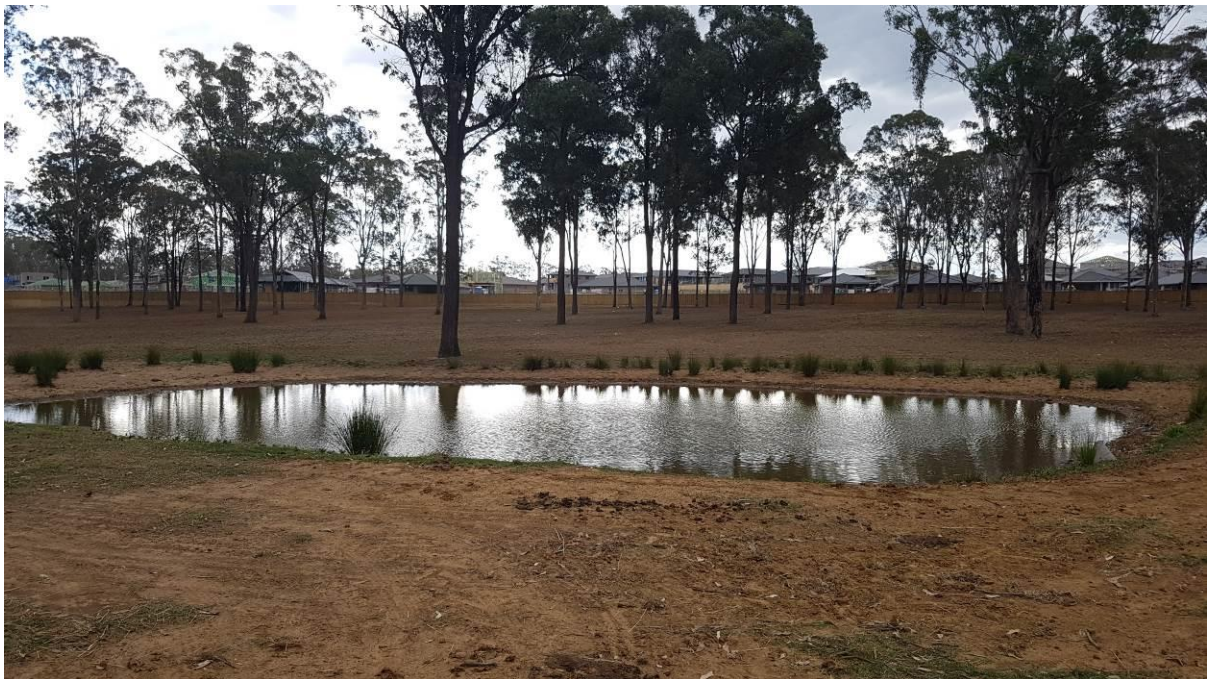
Photo 3-9 – Dam near northern boundary in western portion of the site
